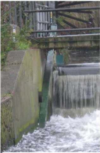
Figure 9 The new eel pass at Ravensbury
