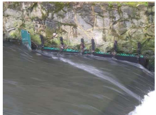
Figure 10 the subsidiary eel pass, showing the bristles used by the eels to push against the water pressure
